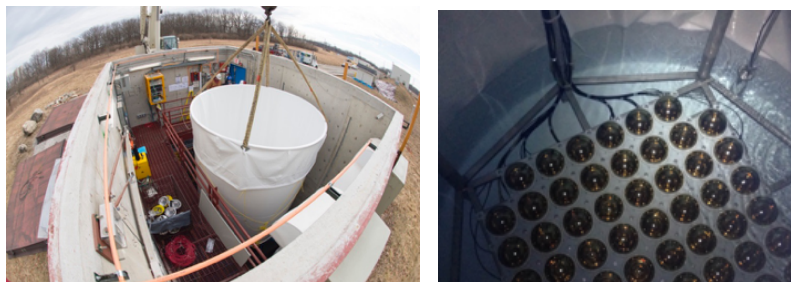
Figure AN-1: Left: The ANNIE water tank being lowered into the experimental hall (formerly SciBooNE). Right: A picture inside the tank, as it was being filled with ultra-pure water.
